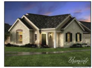
The Bramante—Part of the exciting new Courtyard Collection of floor plans being offered at The Villas at Apple Creek.
